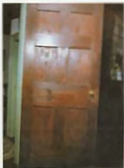
Dining room door, trim and floor pattern
